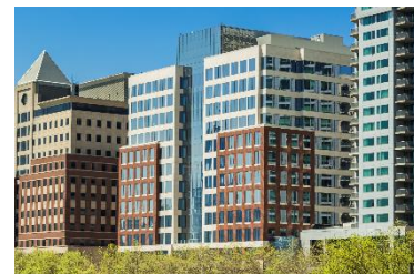
WATERFRONT CORP CENTER III 511,652 SQUARE FEET SJP PROPERTIES HOBOKEN, NJ
